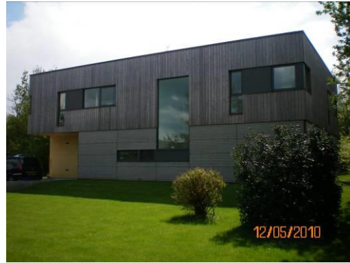
Fig 12: Recently built eco-home at Holly Lodge Farm, Wallington, includes solar panels, passive solar gain, a sedum roof and efficient hot water / heating system.
